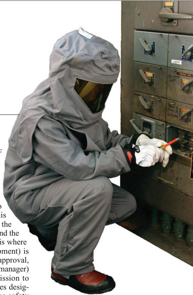
indicating arc flash hazard severity and the required protective equipment should be present at the testing location. If no label exists a qualified engineer must assess what workers need to wear until a complete Arc Flash study is arranged. The following table is a guide:
